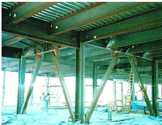
Fig.3.Eccentric brace
